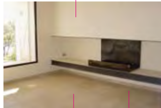
banc béton foyer acier
